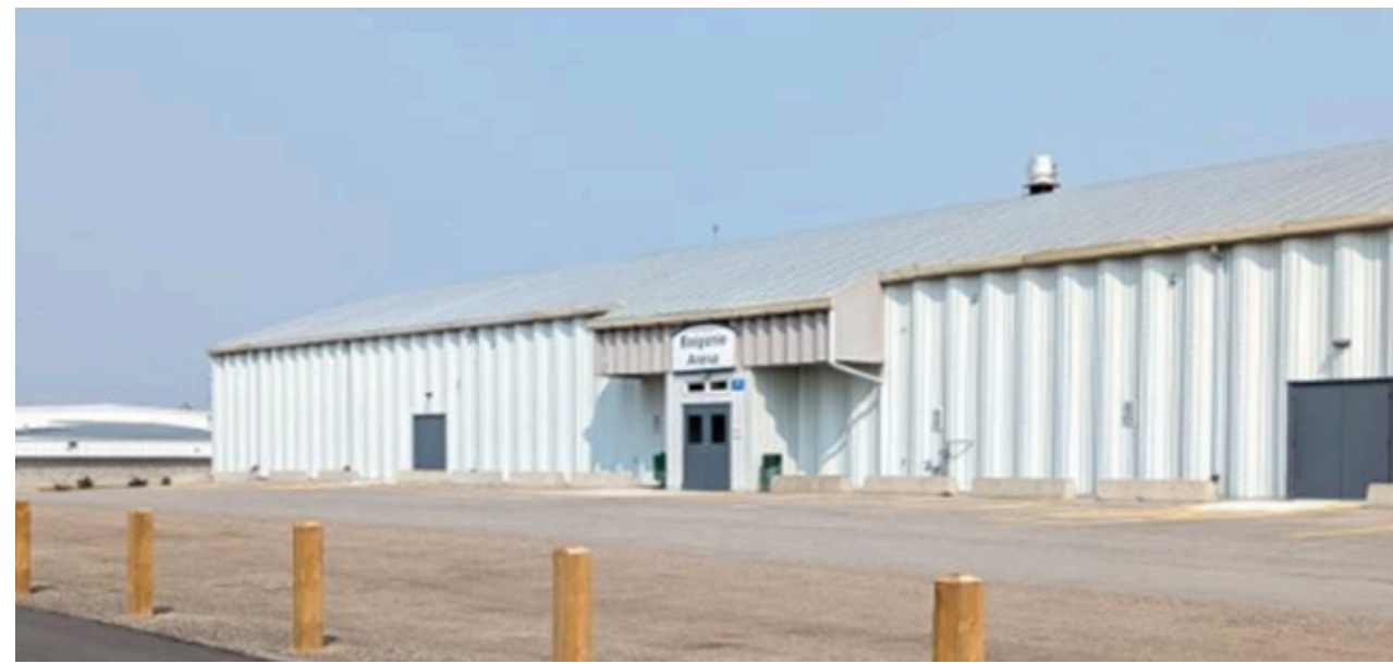
Balgonie Arena (Stardome) - 955 Highway 364
