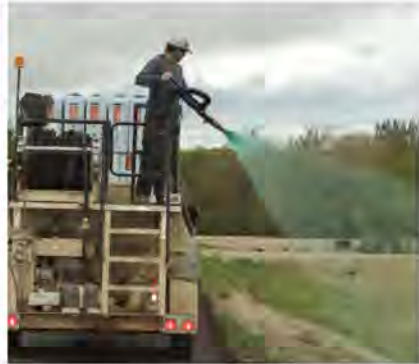
Hydro-seeding by Rapid Lawn at Crawford Developments, August 1.
