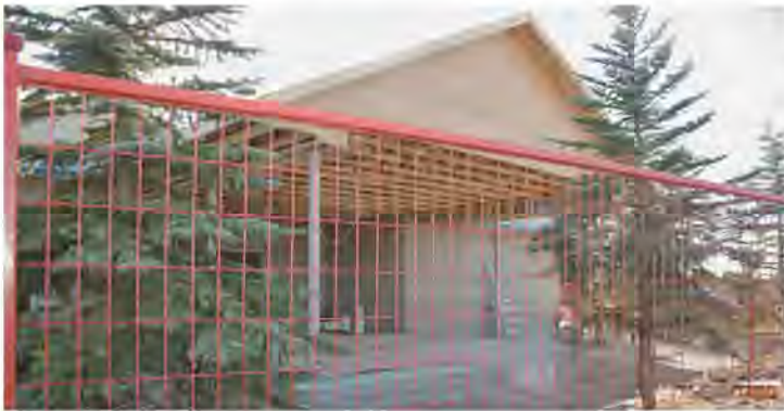
Emerald Park Soccer Centre construction image from October 18.
